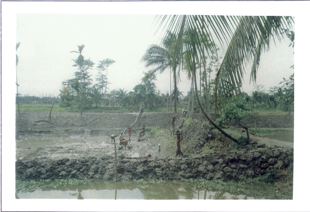
Plate 5.3: Pond construction in progress for scientific fish culture.
