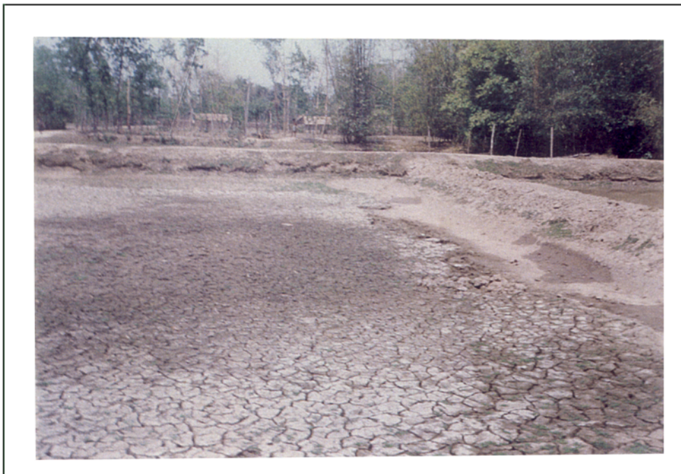
Plate 5.4: Pond preparation and strengthening embankment.
