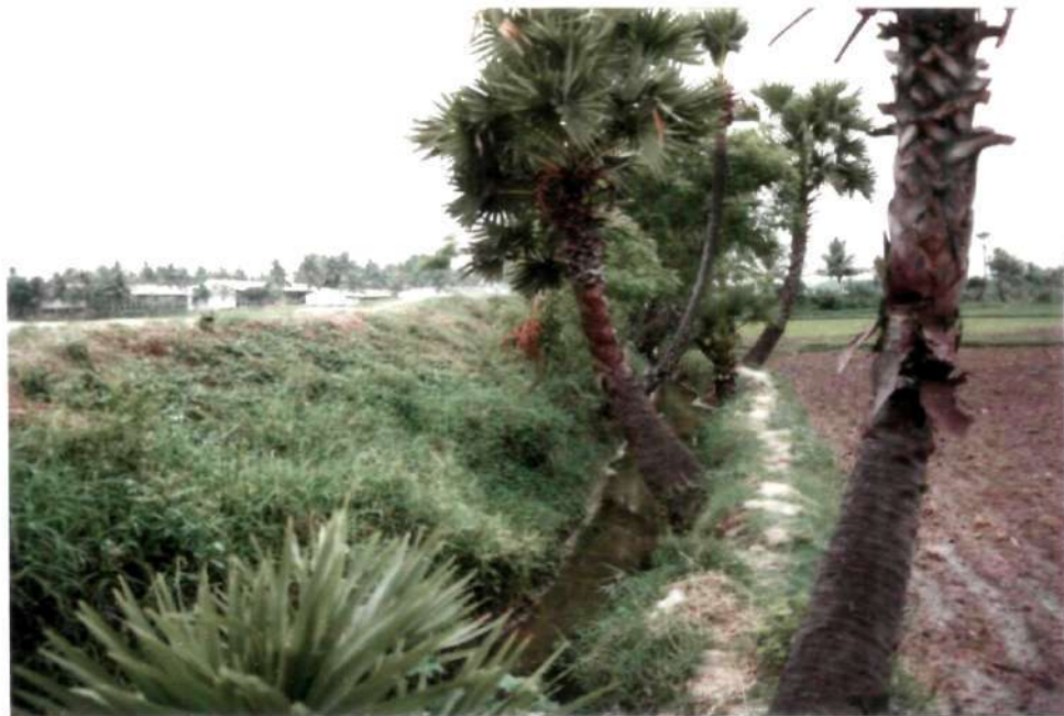
Plate 4: Location of the drainage channel by the side of the fish pond at Rebala
