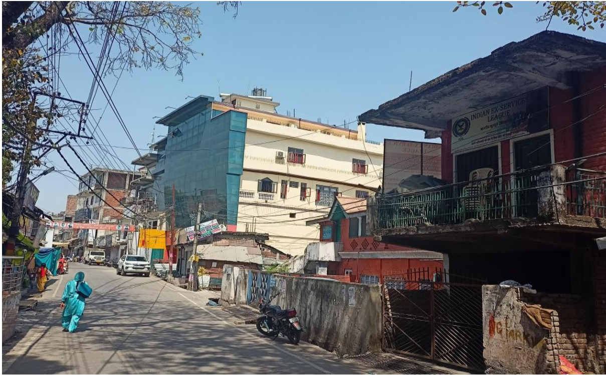
Fig. 4.7: Ground truthing points of built-up area of Hamirpur block, ( 31°41'7.45"N, 76°31'24.03"E)
