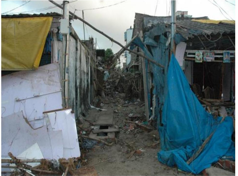
Plate 22. Telephone lines damaged by Tsunami
