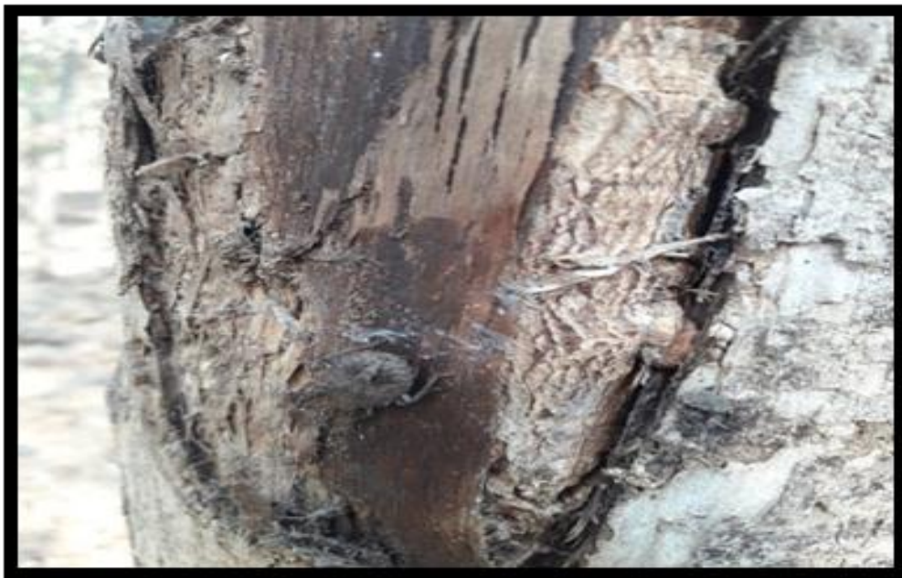
Plate 8.2: Nature of damage
