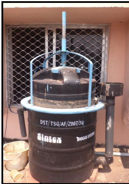
Fig. 4.9 (a) Biogas plant
