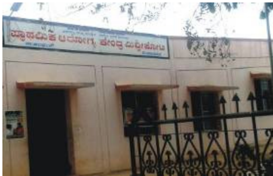
Plate 2: PHC at Mishrikoti, Kalaghatgi
