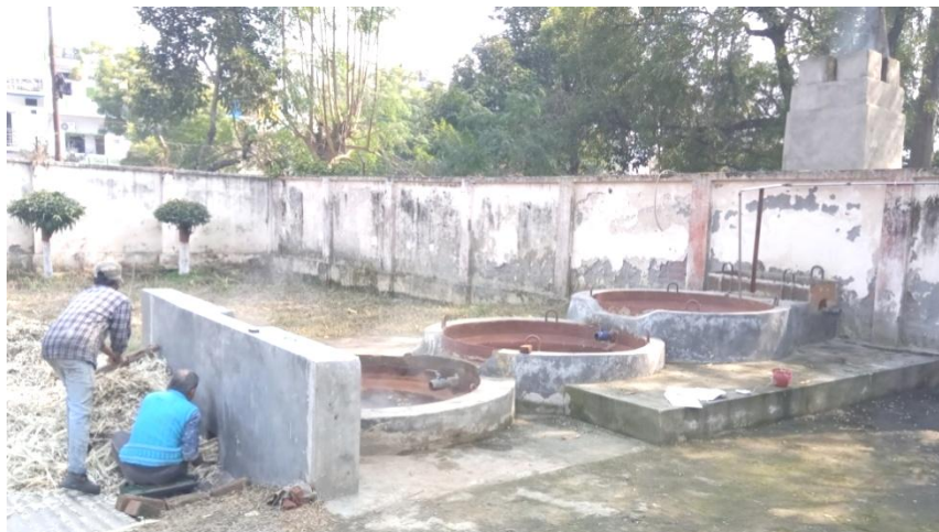
Fig 3.3: IISR three pan furnace
