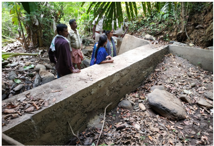
Check dams to control water runoff
