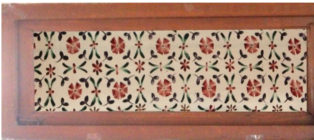
Figure 3.85. Painted roofing II.
