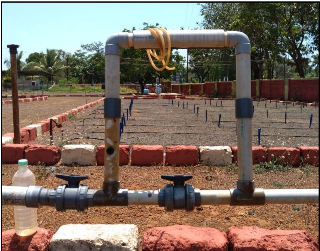
Plate 3.24 Schematic picture and view of developed device for fertigation
