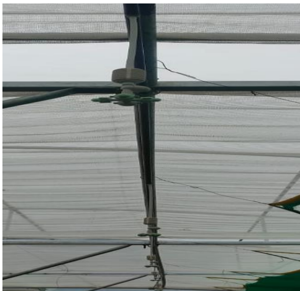
Plate 3.5 Foggers used in the naturally ventilated polyhouse
