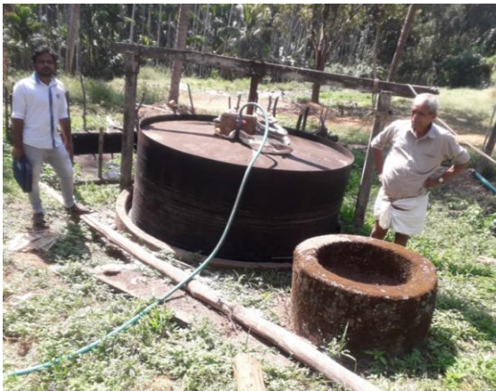
Plate 4: Exchanging information with the biogas plant owner
