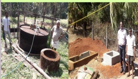
Plate: 1. Floating and Decnabandu type of biogas plant
