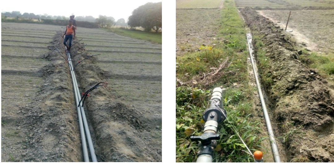
Fig. 3.4: Drip system installation at field
