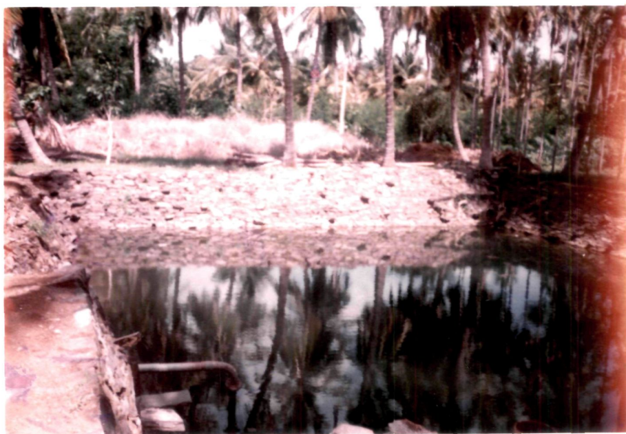
Fig6: Water storage structure in one of the farms in Hiriyyur
