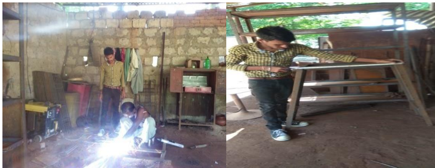
Fig 3.7: Fabrication work in the workshop
