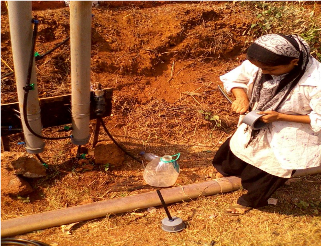
Fig. 4.15 Fitting of air vent to end cap
