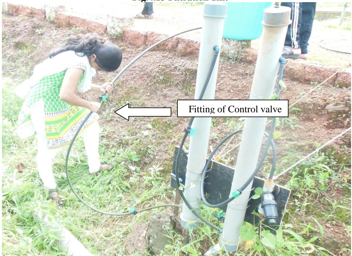
Fig. 4.14 Fitting of control valve
