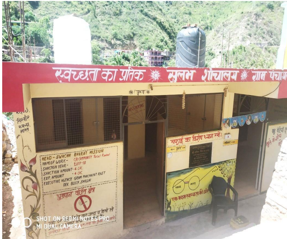
Fig 4.7 Community toilets constructed by panchayat Shillai under Swacch Bharat Mission
