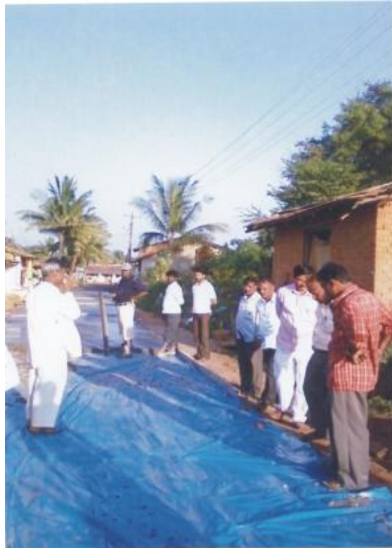
Plate 2. Construction of panchayat building
