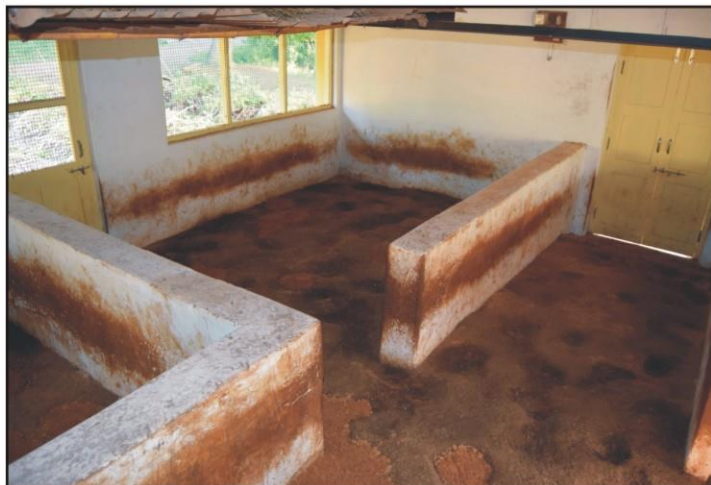
Plate 6: Internal view of sheep house
