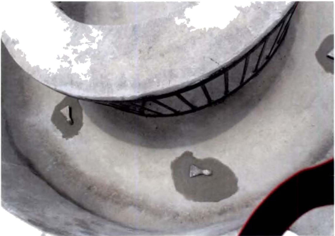
Plate:17 Modified design of inlet in the hatching pool for better flow rate in a govt. Hatchery.
