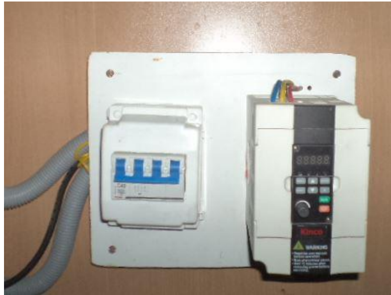
Plate 3. Variable Frequency Drive used for varying the roller speed of Aloe vera gel extraction machine
