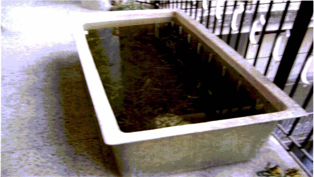
3. Water storage tank
