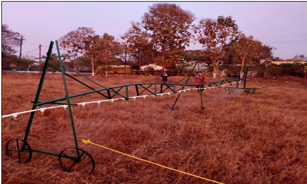
Fig 3.14 Actual view of boom support span
