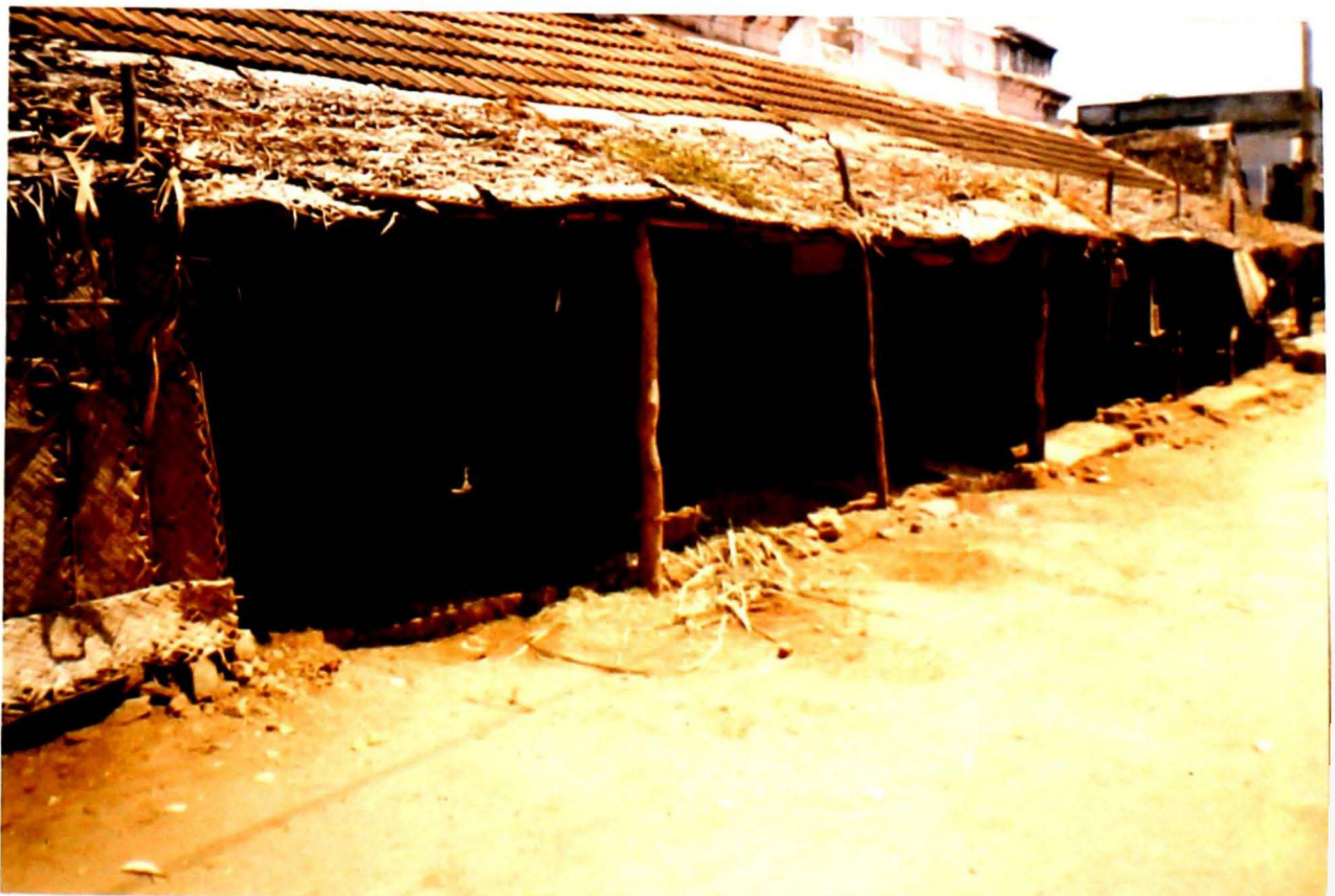
Plate No. 2. A view of front portion of house partly being used as cattle shed
