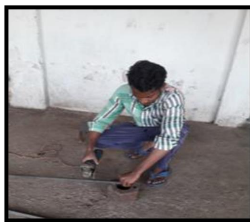
Plate 3.14 Cutting of the plate and rods
