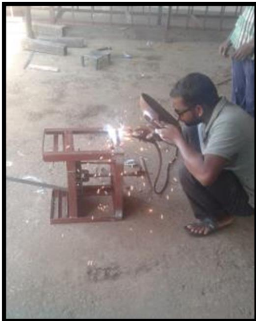
Plate 3.17: Welding process during fabrication
