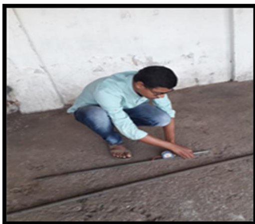
Plate 3.13 Marking the rods for cutting
