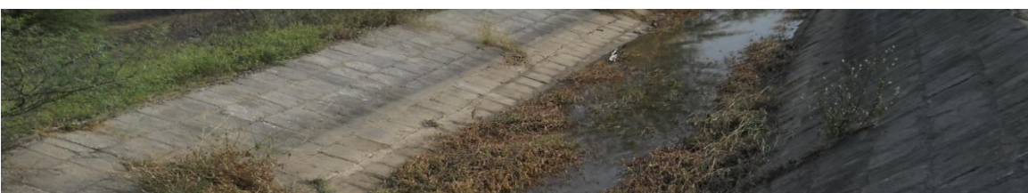
Plate 4: Silt measurement in Right Main Canal at CH 415
