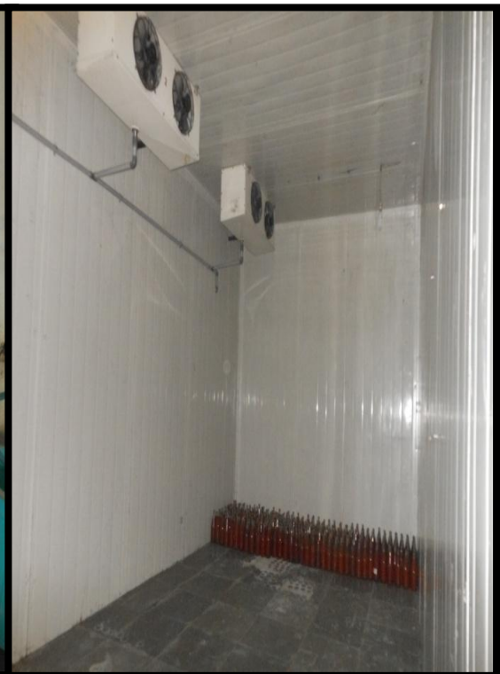
Plate 3.16 Cold Storage Room
