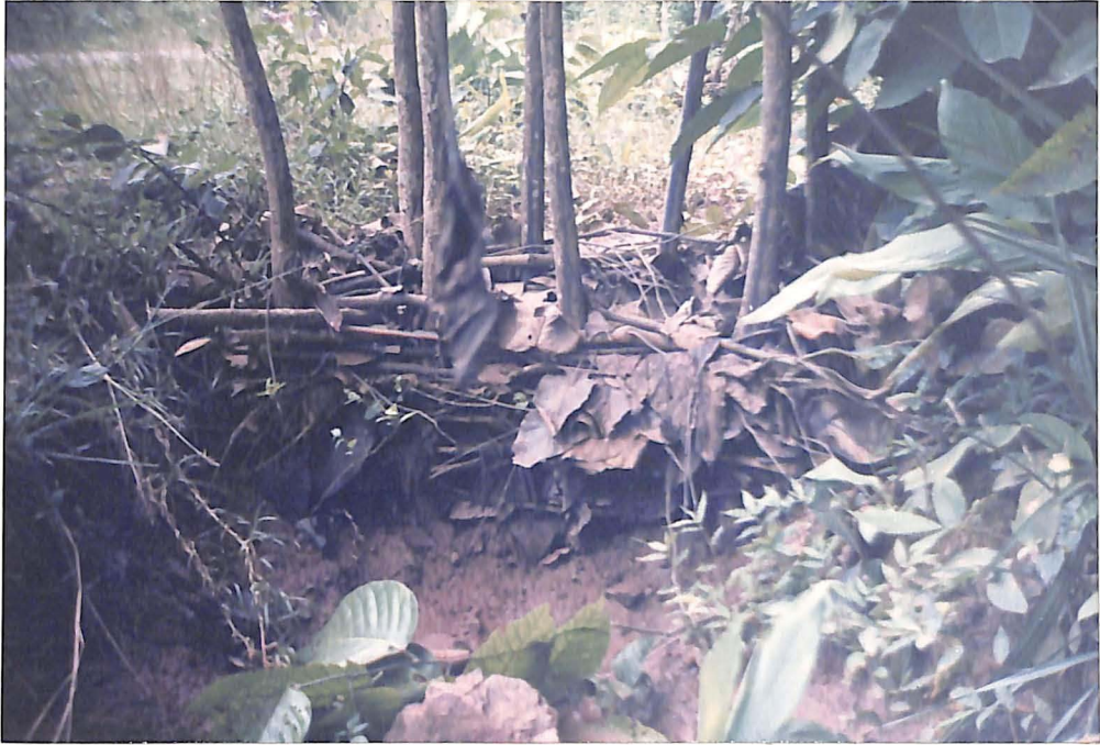
Plate No. 1 Brushwood structure across gully
