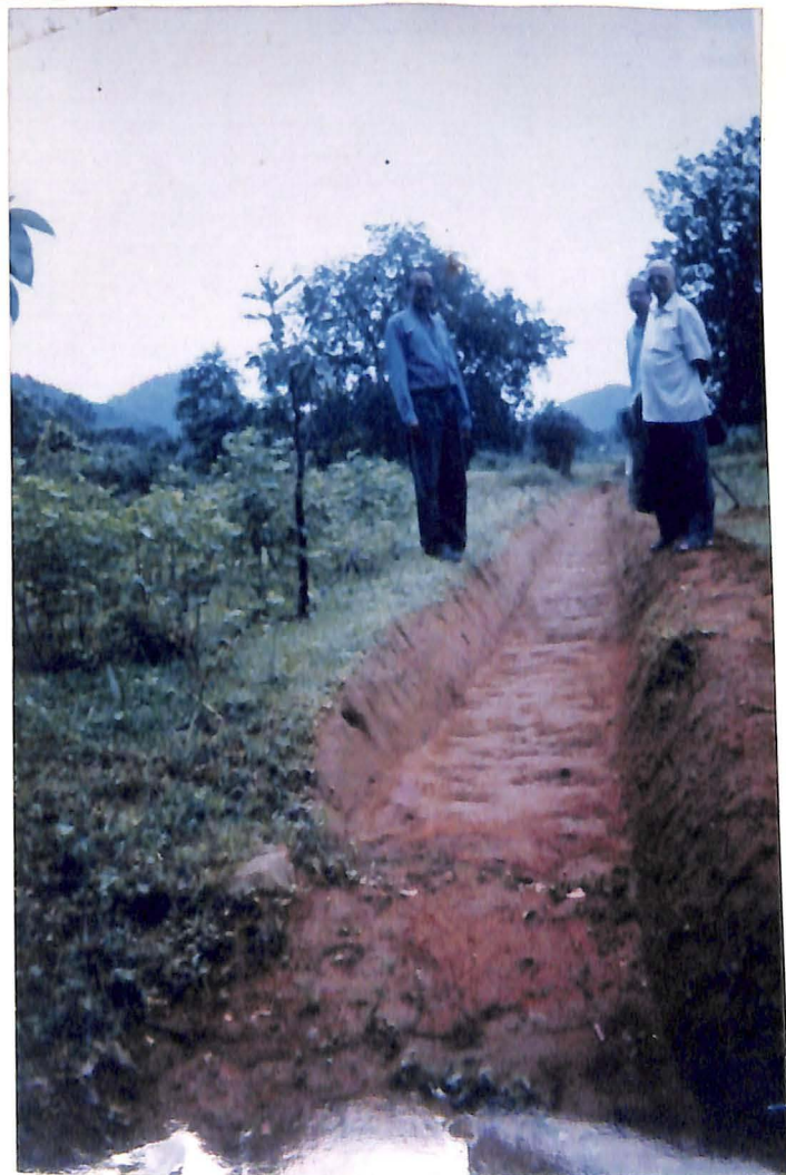
Plate No. 8 Diversion drain for intercepting run
