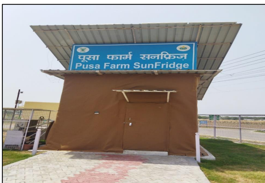
Plate 3.3. Pusa Farm Sun Fridge constructed at mela ground, IARI
