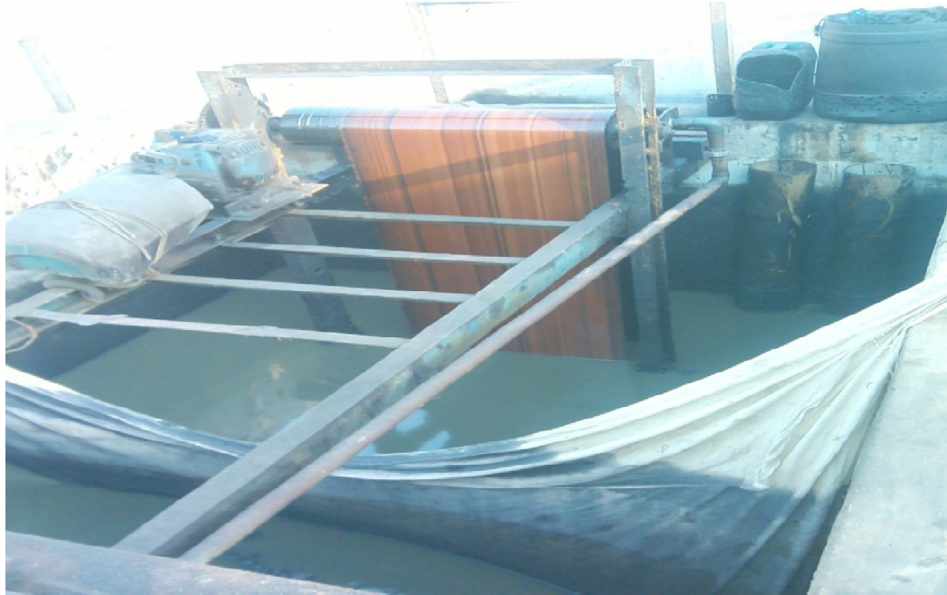
Fig. 15: Skimmer belt- separations of oil and chemicals from waste water
