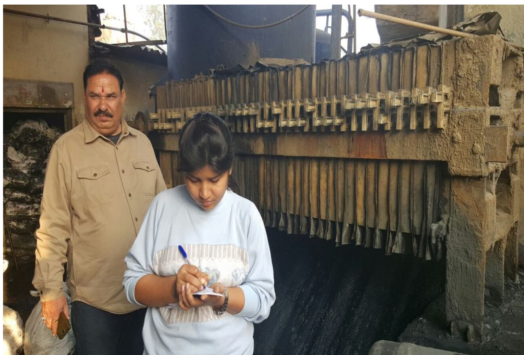
Fig. 23: Waste effluent compressor
