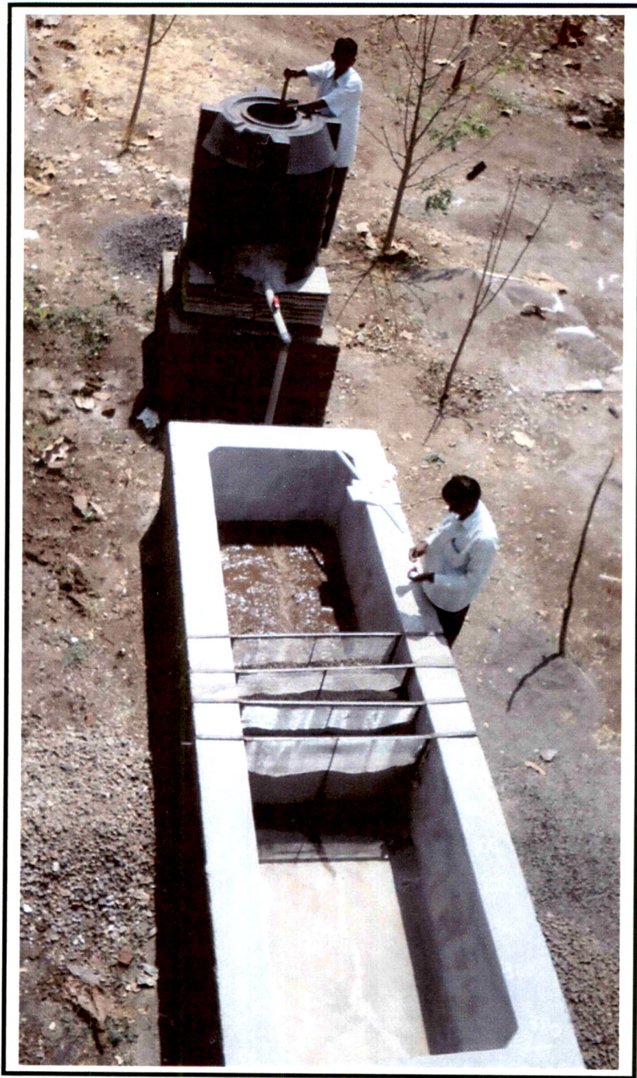
Plate 7 : Measurement of time of filtration
