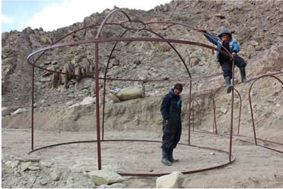
Plate 3.2: Making of iron dome
