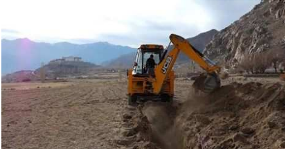
Plate 3.1: Mechanical excavation for source pipe line
