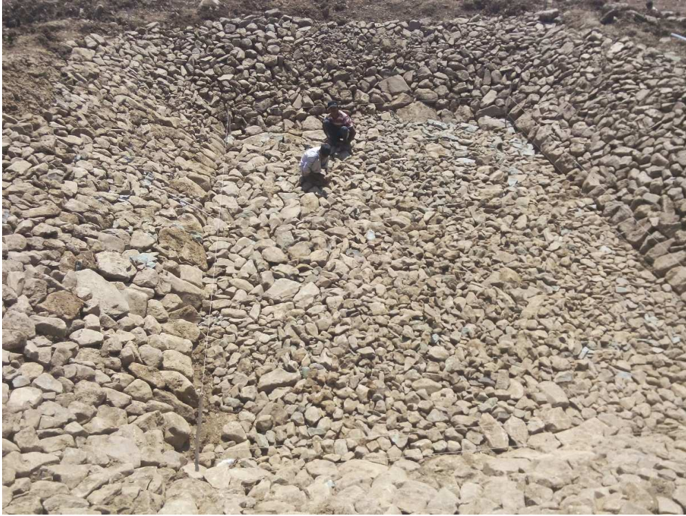
Plate 4.4: Construction of R.C.C Tank
