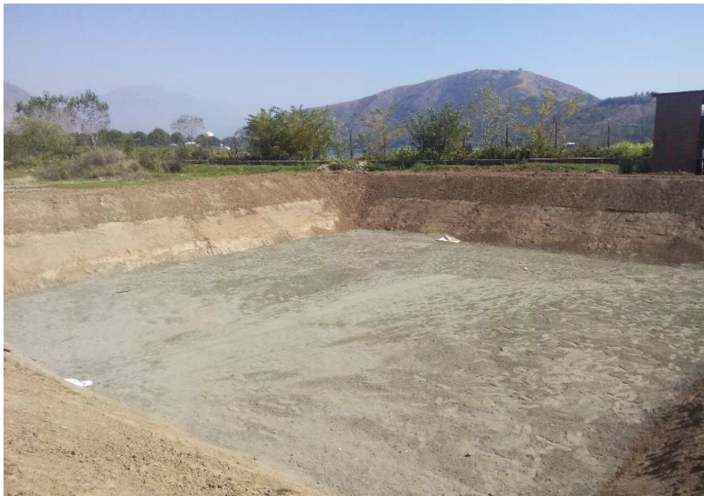
Plate 4.2: Under construction earthen pond
