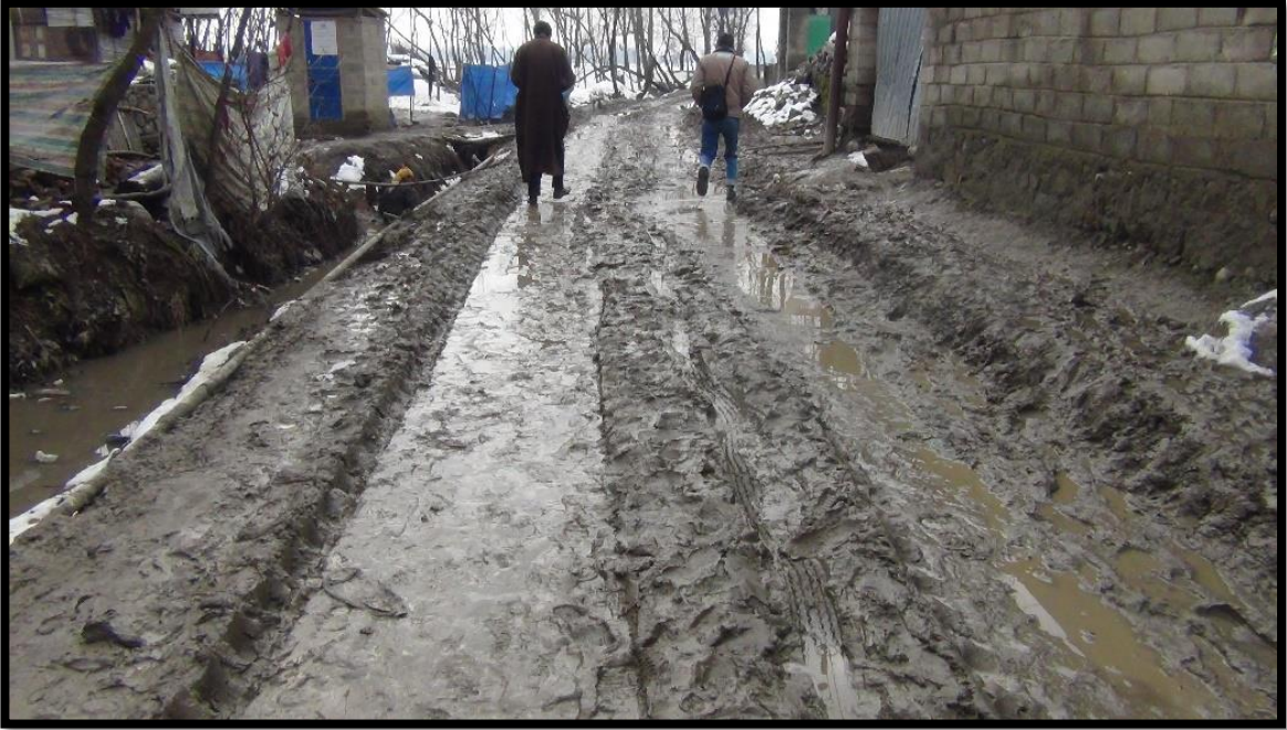
Plate 5: Bad road leading to Laharwalpora landing center
