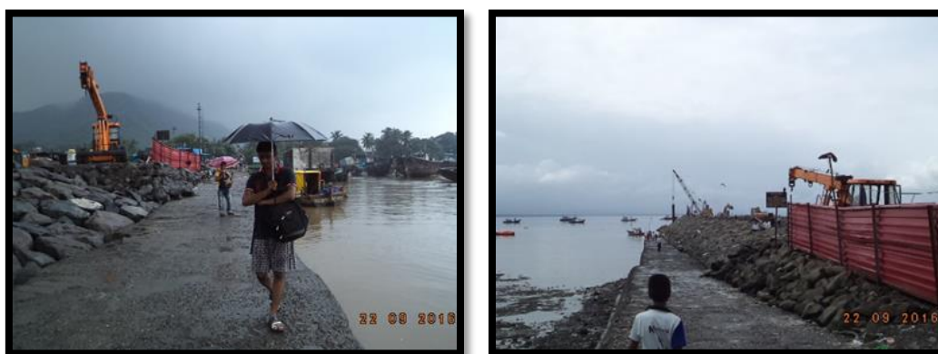
Fig. 4: Wharf of Karanja with upcoming constructions
