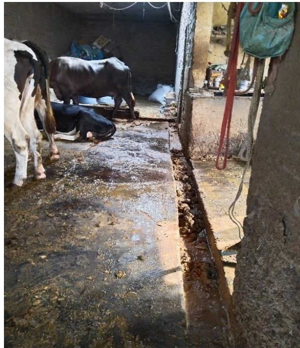
Plate 4.2 (c): Poor drainage
