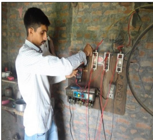
Fig. 3.3e. Measurement of electrical parameters
