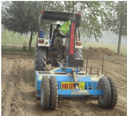
Fig. 3.7c. Laser guided land levelling
