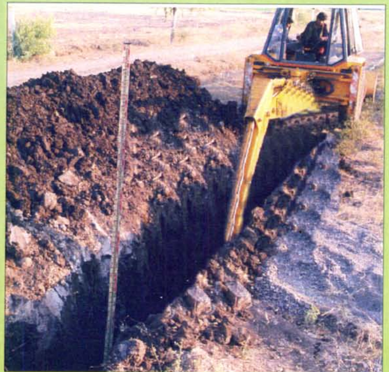
D) Excavation of trench for laying drainage pipe
