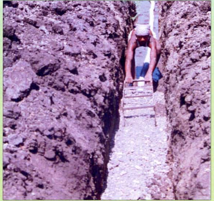
B) Covering of drain Pipe with Sand
