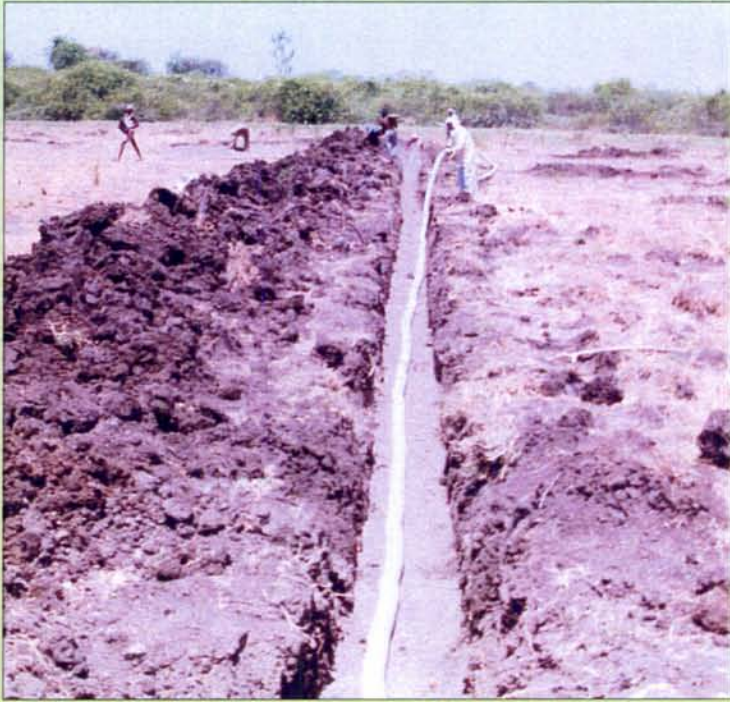
A) Laying of drain Pipe
