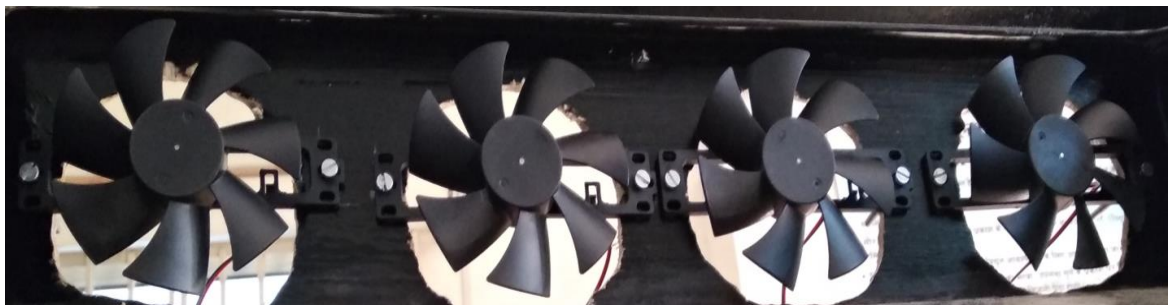
Fig. 3.10 Installation of DC fans at duct exit
