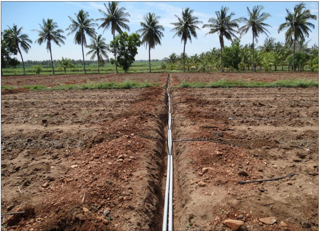
Plate 2: Drip system installation
