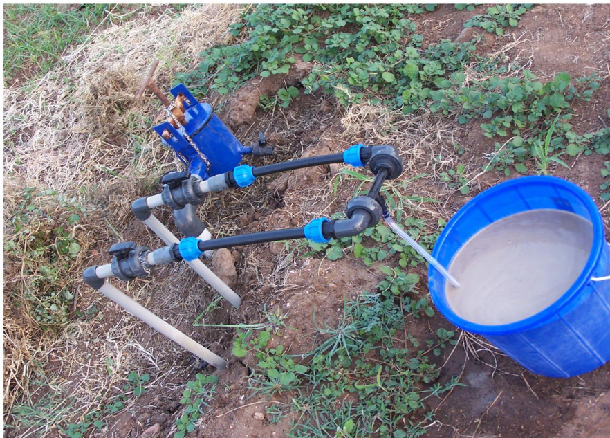
Plate 4. Fertigation through venturi system
