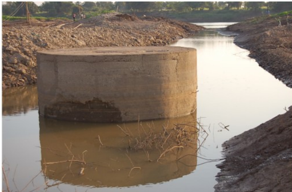
Plate 8. A close up of intake well
