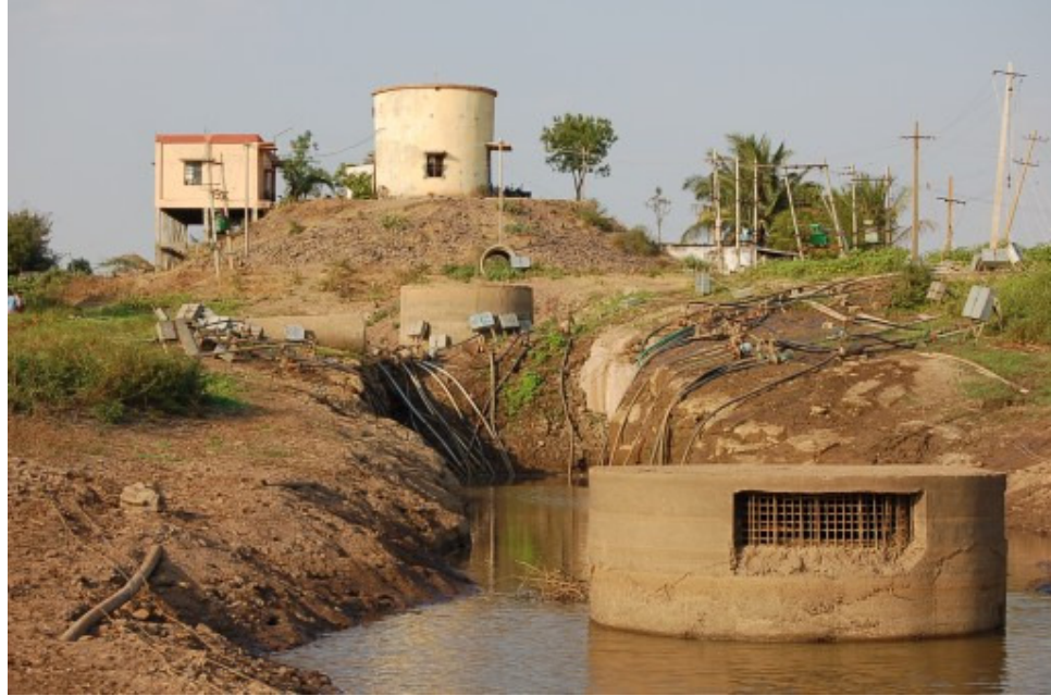
Plate 7. Water is lifted from the intake well in the river (power house in the background)
