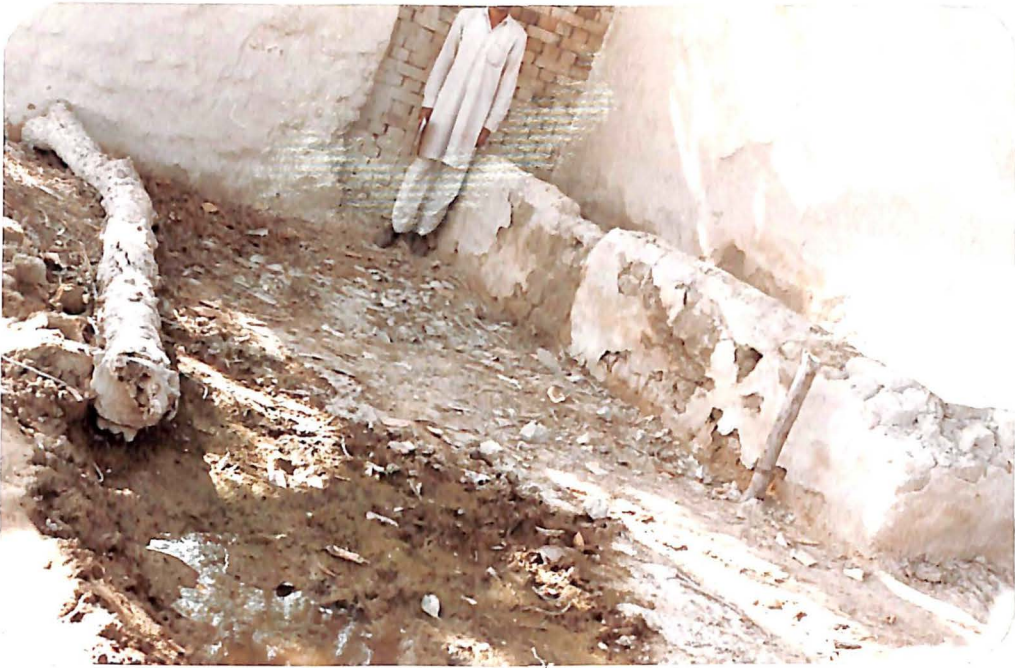
Fig. 11. Dirt floor with uneven surface, no drainage and dirty. Mangers made of mud.
