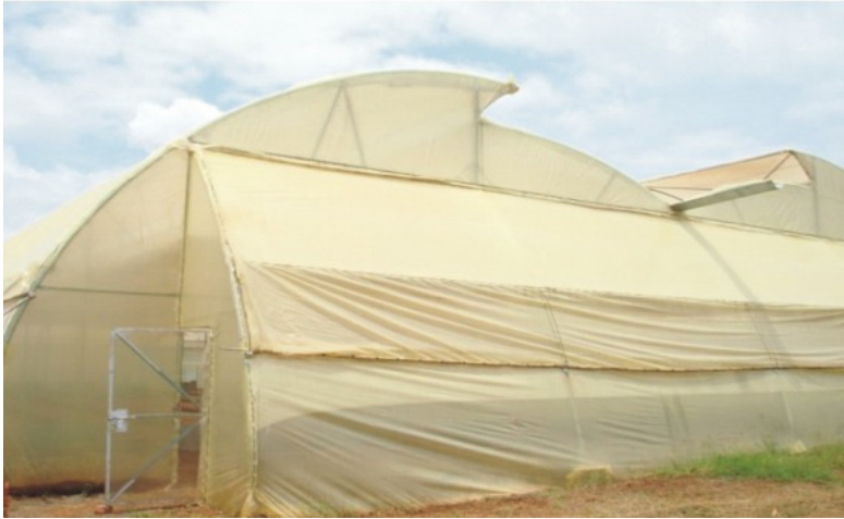
Naturally ventilated poly house
