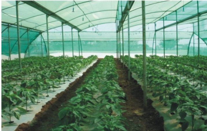
Naturally ventilated poly house
