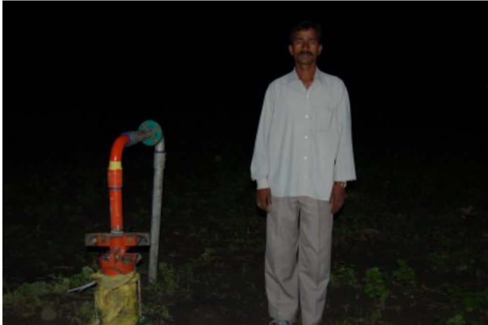
Plate 11. Failure of bore well due to wrong choice of the site
