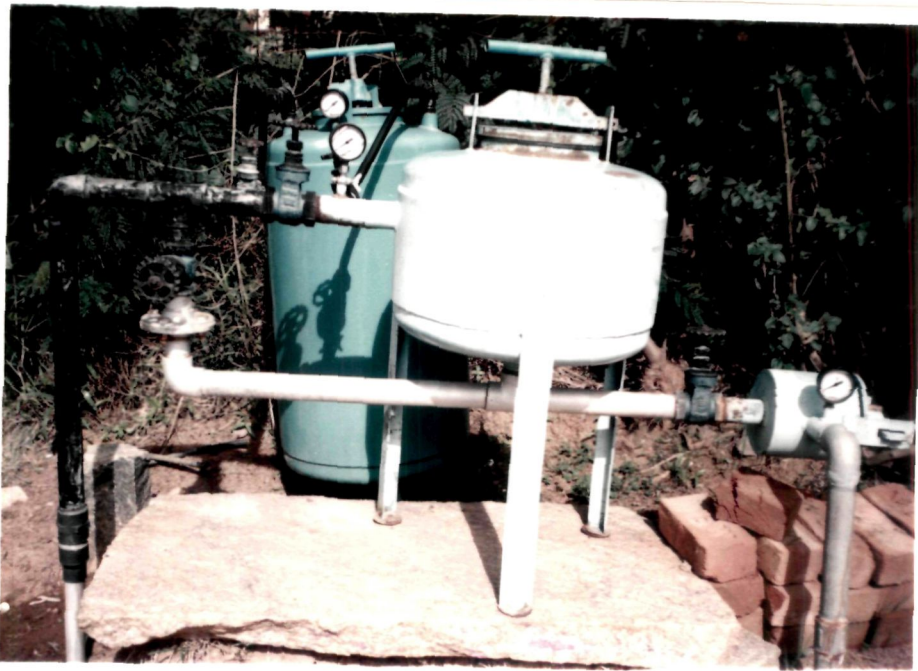
Plate 3.3 - Fertigation tank with sand and mesh filters
