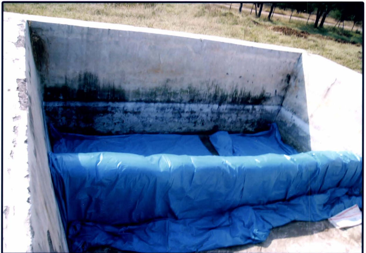
Plate 2. Concrete trench silo pit, which was used for urea treatment of sugarcane tops.
