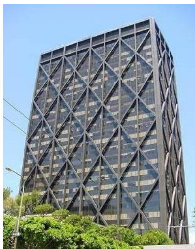
Fig. 1.6 Building with steel bracings
