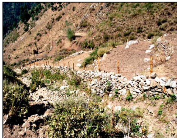
Stream Bank Stabilization at Dara
