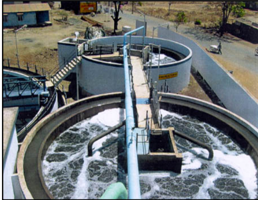
Sewage Treatment Plant at Nishat
