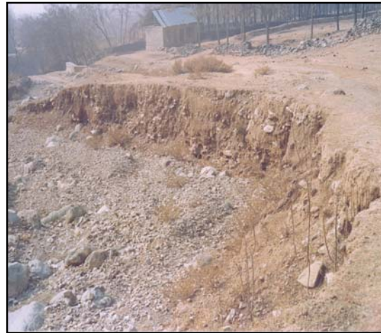
Stream Bank Erosion
