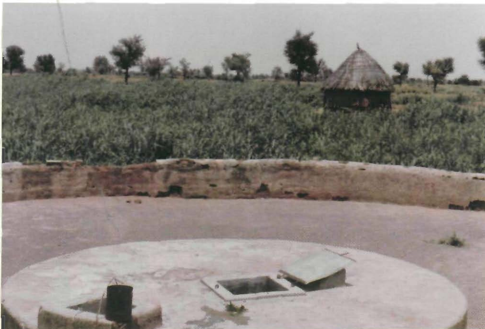
Rain water harvesting
