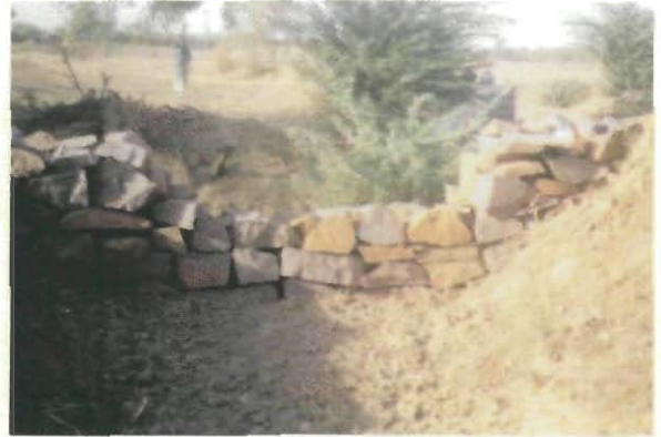
Gully plugging with rocks/stone
